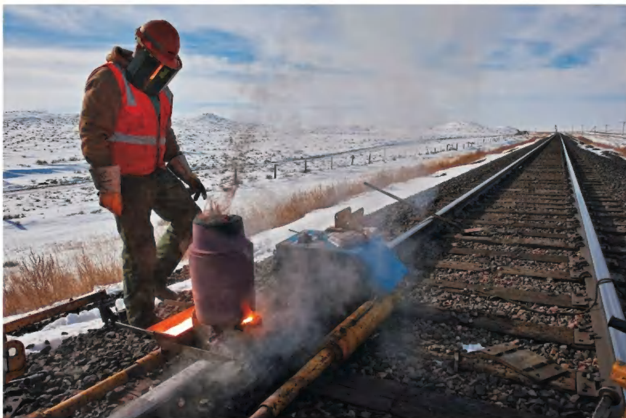
Justin Hofeldt, a welder for BNSF Railway, repairs track near Rudyard. The rails opened this ground to homesteaders, with illusory promises of easy crops and plenty of rain.
